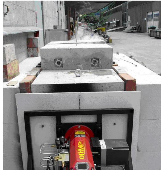
Fig. 5. Gas heater OLYMP 3520 and escaping water
