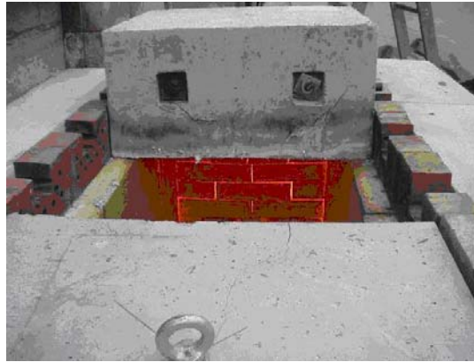
Fig. 3. Furnace with a typical FRC block.
